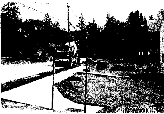
Sidewalk Replacement in Atlanta
